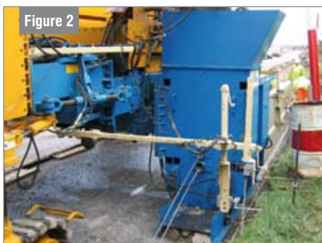
Wire strands feeding through mould
