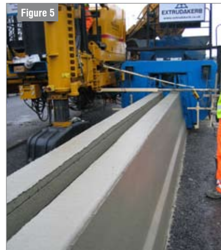
Paving Trough Variable Wide Concrete Step Barrier
