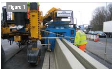
Wide Variable CSB with integral cable trough
