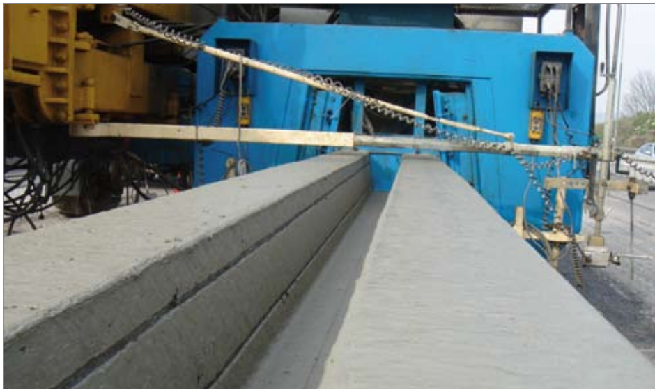
Wide variable CSB with integral cable trough
