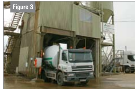
Figure 3 Dedicated concrete plant
